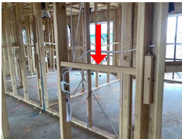
FIGURE 6.3 TYPICAL WALL JUNCTIONS
