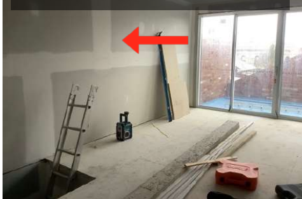
TV area, out by 12 mm over 1.8 m, vertically
