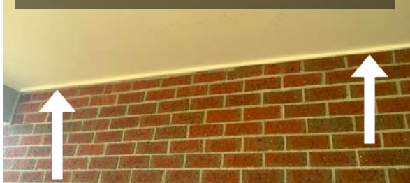
The bed joint is not running horizontally straight, you can see that the alfresco ceiling has the bed joint fully exposed of over 10 mm at one end and at the other end the bed joint is completely hidden
