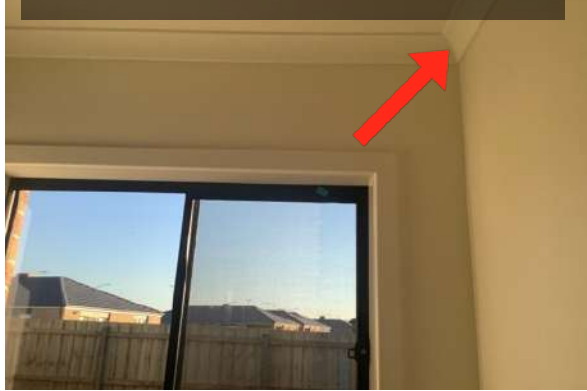
Excessive cornice junction in bathroom
