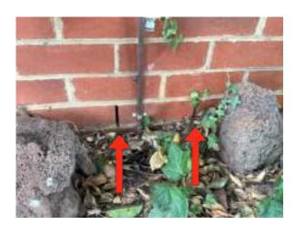
UNTREATED OR NON-DURABLE TIMBER USED IN A HAZARDOUS ENVIRONMENT
